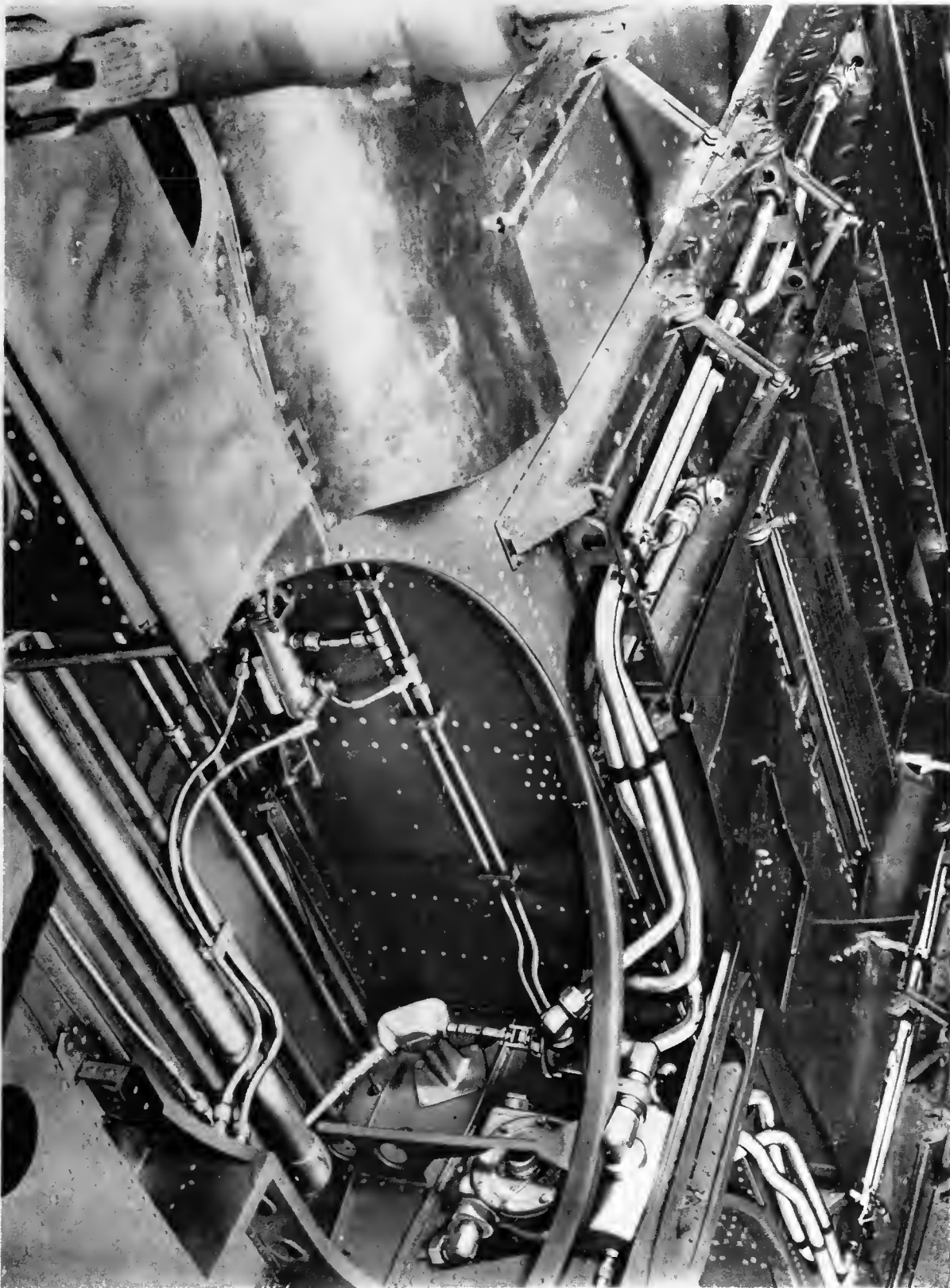
8266 - Fuel Lines Installation
